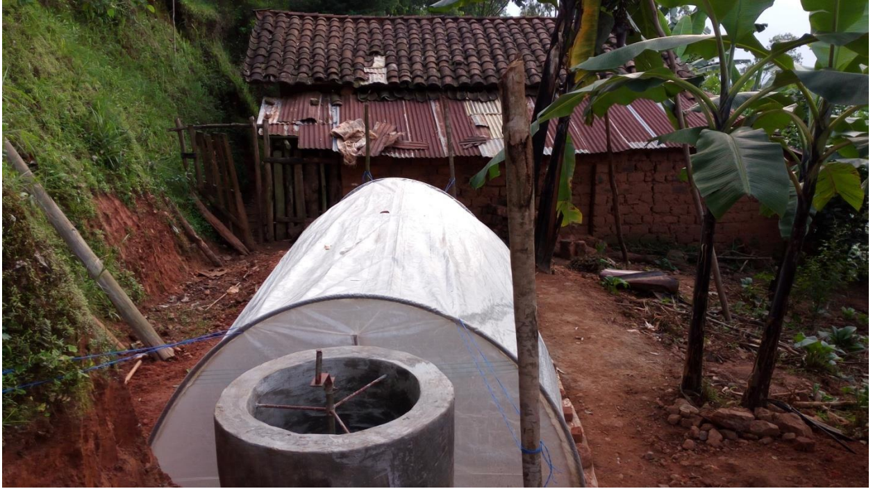
Fig: Complete Canvas biogas systems installed at the youth piggery cooperative.
