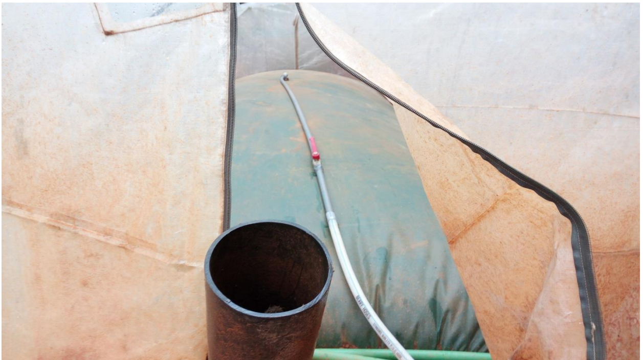
Fig 2: An inflated biogas digester after completion of the initial loading
